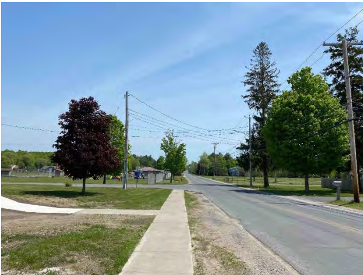
Existing Sidewalk on Maple Street looking east
