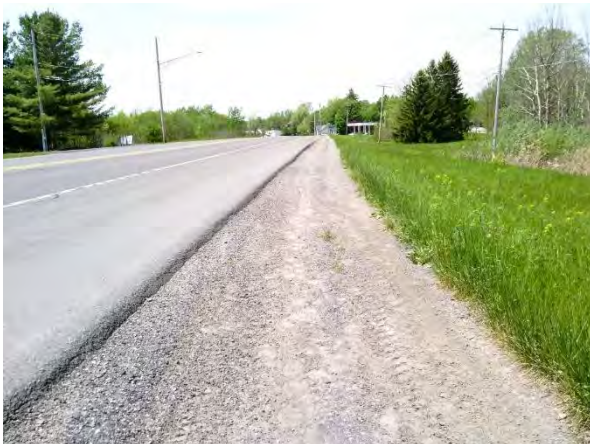
Shoulder area within Segment A
