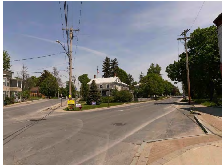
Intersection of North Main Street, Maple Street, and Leray Street.
