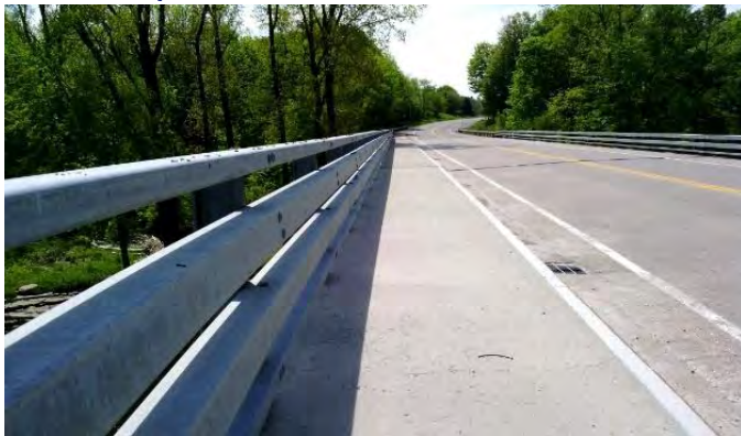
Bridge over Route 971V
