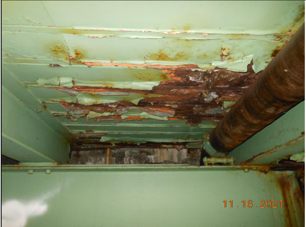
Photo Number: 1 Photo Filename: 01_Underside of Deck in Stringer Bay 1 above
