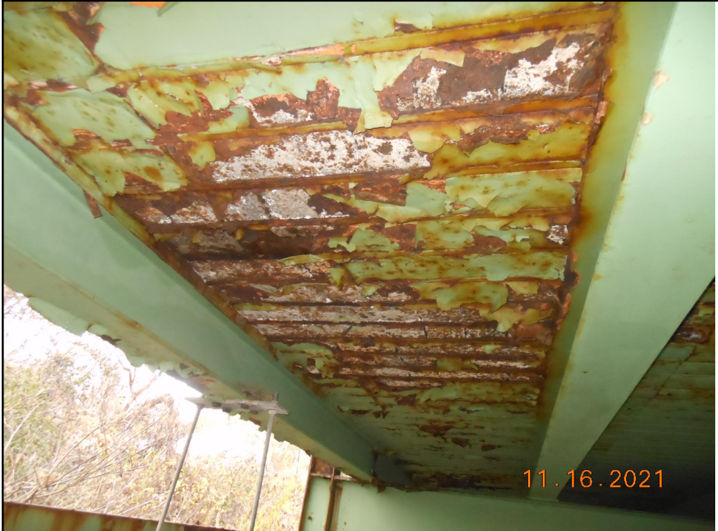
Photo Number: 2 Photo Filename: 02_Underside Of Deck In Stringer Bay 4
