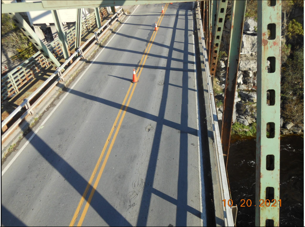
Photo Number: 11 Photo Filename: 11_Wearing Surface at the End Half of Span
