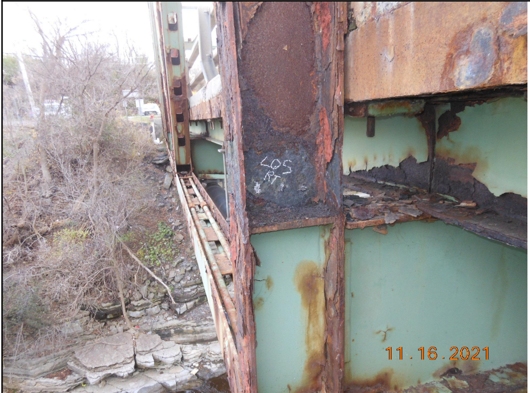
Photo Number: 16 Photo Filename: 16_End Face of Right Truss Vertical Member
