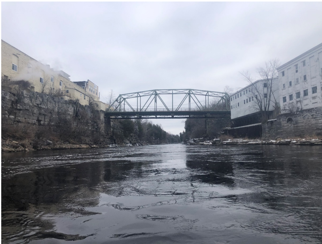
Recent Photo Looking Upstream During Lower Water Levels
