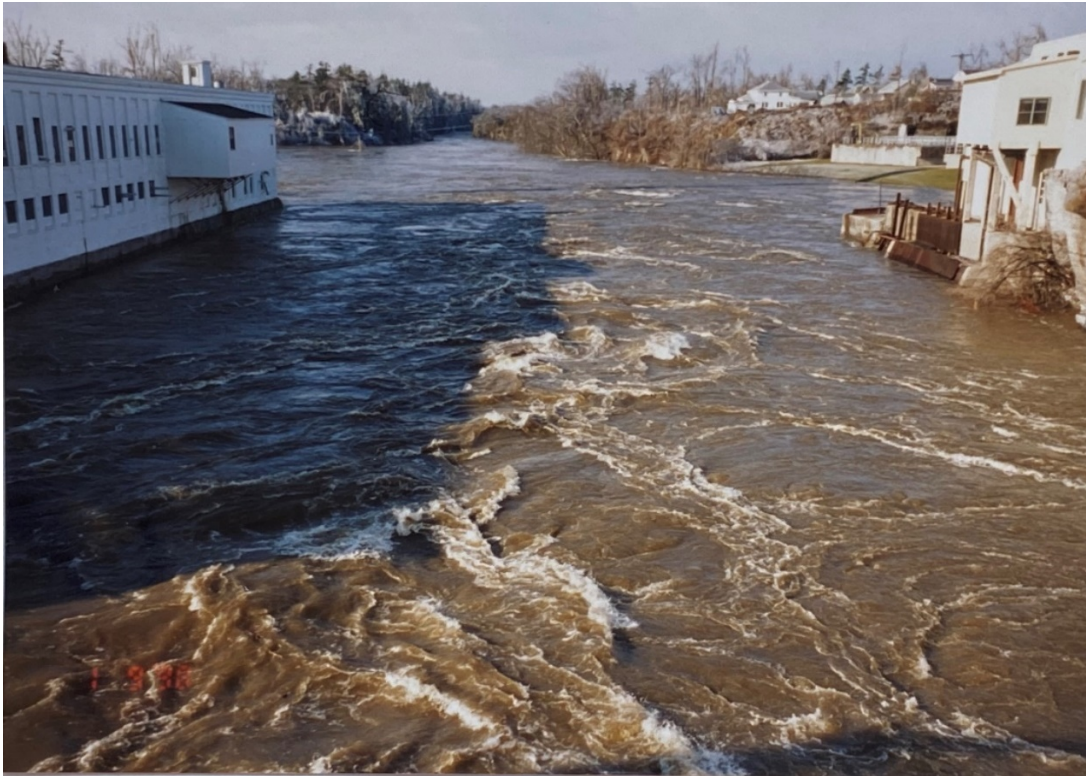
Looking Downstream – From BIN 3338900 Jan. 9 th , 1998
